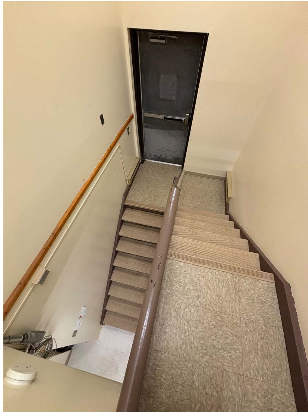
The basement stairs to programming space. Also the basement has the only storage for staff supplies; i.e. crafting materials and programming equipment.
