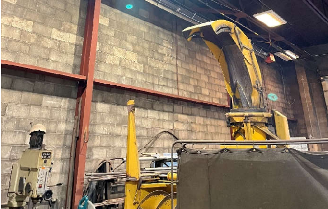
Figure 45: Typical Garage Uninsulated Concrete Block Wall
