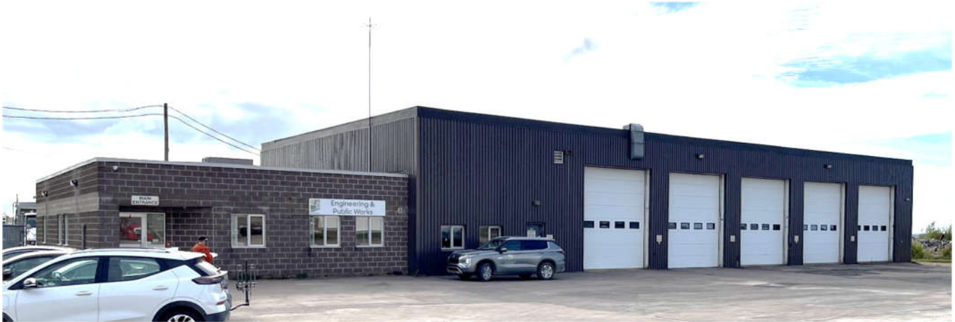
Figure 3: Tantramar Public Works Depot, Sackville NB
