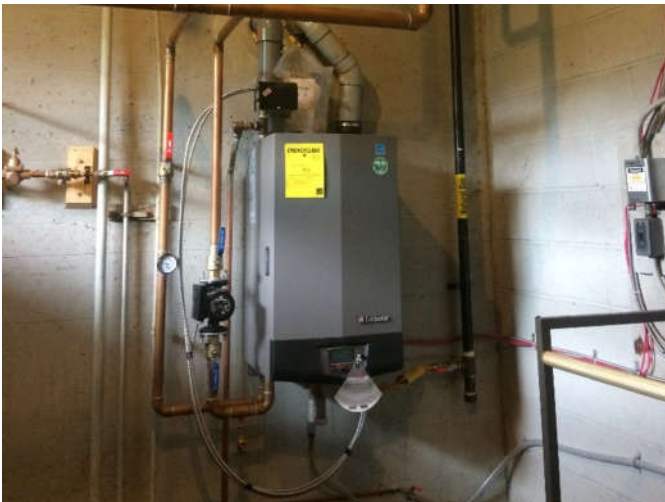
Figure 38: Lochinvar Condensing Natural Gas Boiler
