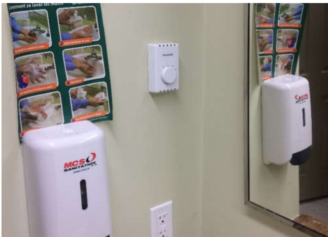
Figure 41: Typical Line Voltage Thermostat
