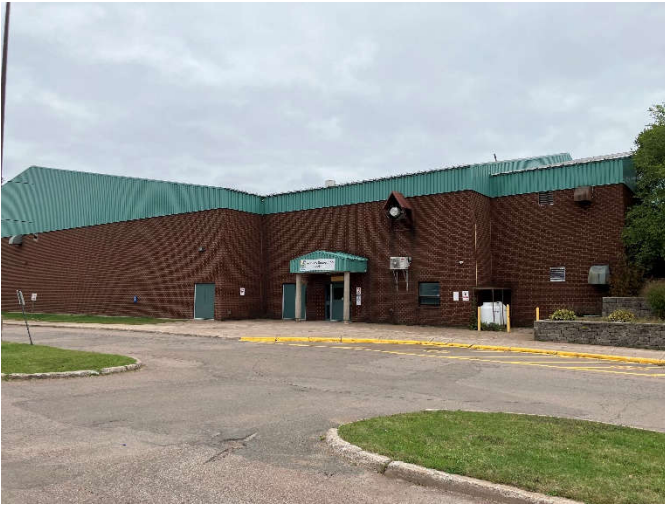
Figure 10: Brick Exterior Walls
