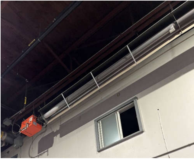
Figure 52: Typical Infrared Tube Heater
