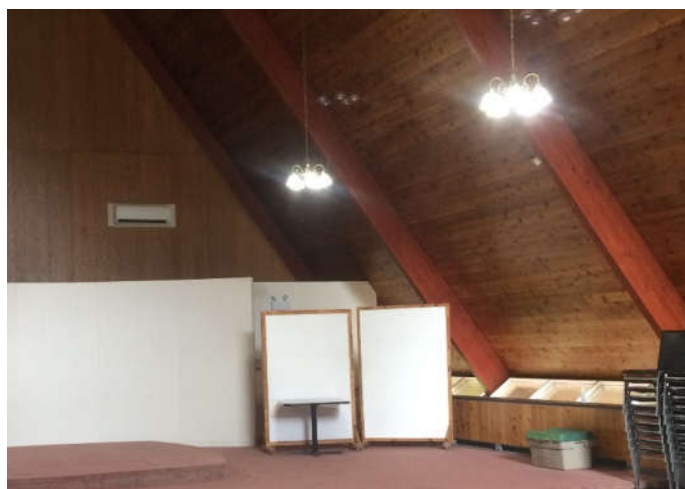
Figure 43: Typical Main Level LED Lighting (LED Screw-in Bulbs)
