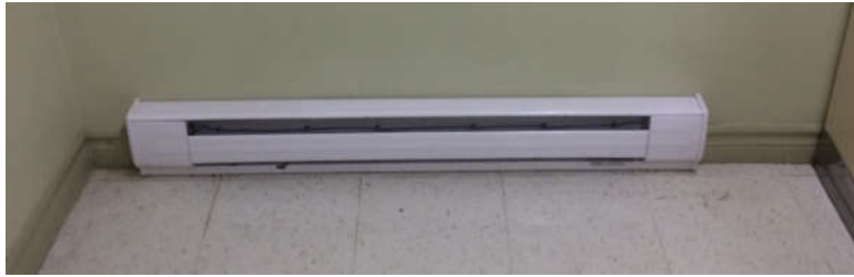
Figure 40: Typical Electric Baseboard
