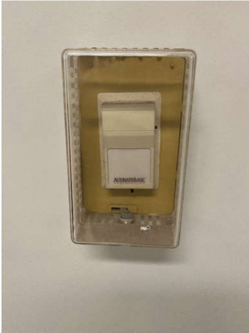
Figure 25: Typical Automated Logic Temperature Sensor
