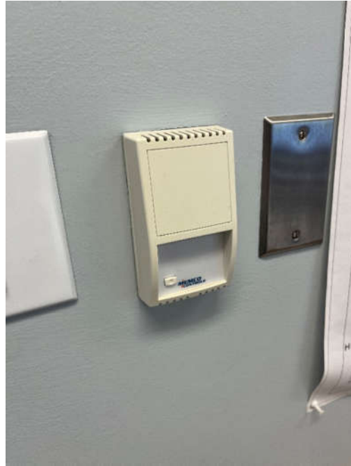
Figure 57: Typical Automated Logic DDC Temperature Sensor
