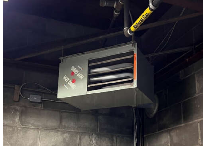
Figure 53: Typical Gas-fired Unit Heater
