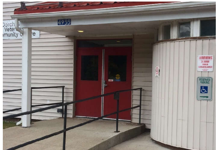
Figure 35: Typical Exterior Door
