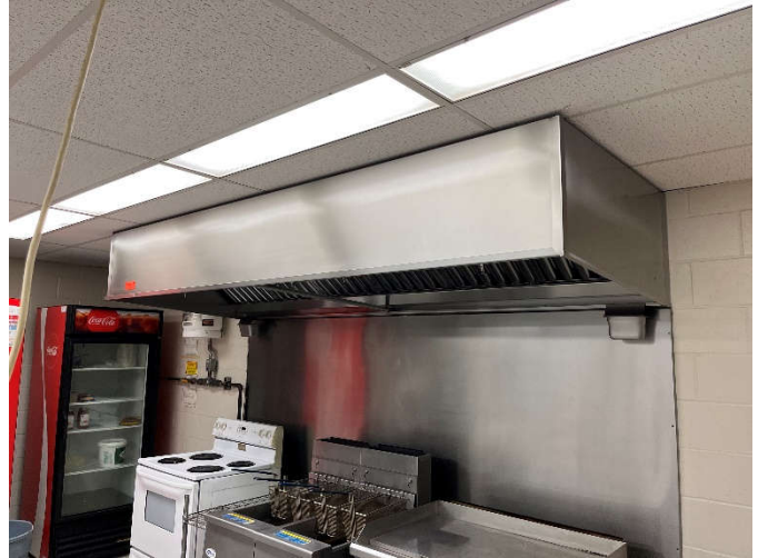
Figure 19: Canteen Kitchen Grease Hood
