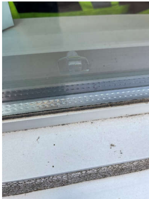
Figure 51: Typical Administration Area Aluminum-Frame Window
