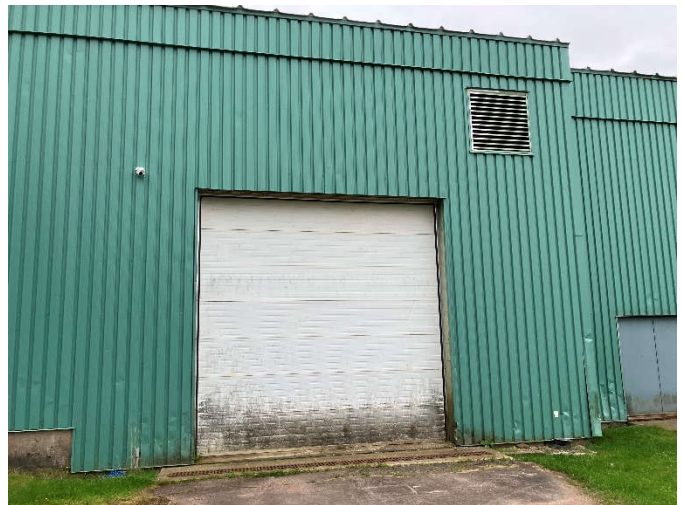
Figure 13: Ice Resurfacers Overhead Door and Metal Siding Exterior
