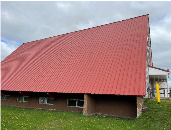
Figure 34: Building Roof and Basement Foundation
