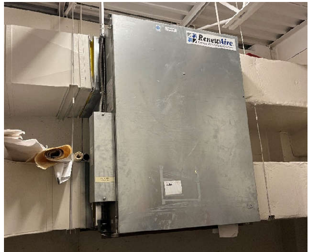
Figure 15: Typical RenewAire Air Exchanger
