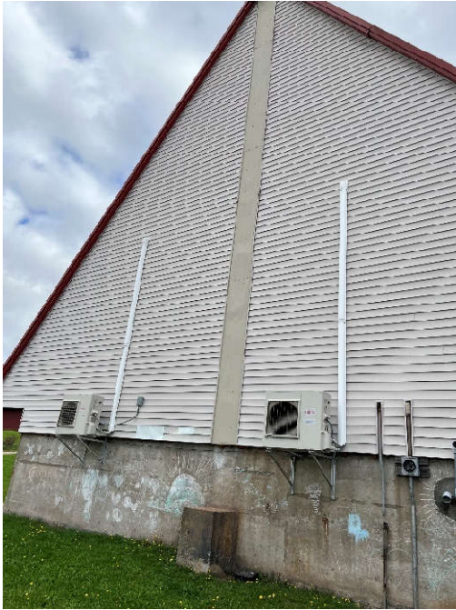
Figure 32: Exterior Wall Siding
